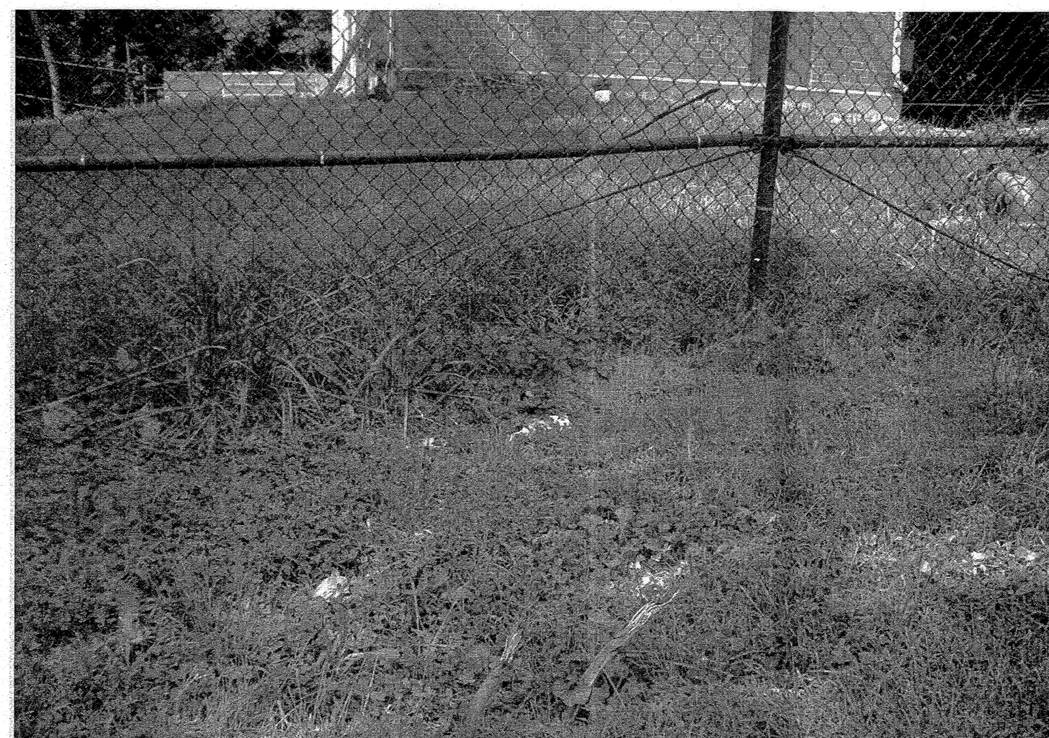
5 D-2 ELECTRICAL FEEDERS AND FENCING ①②
