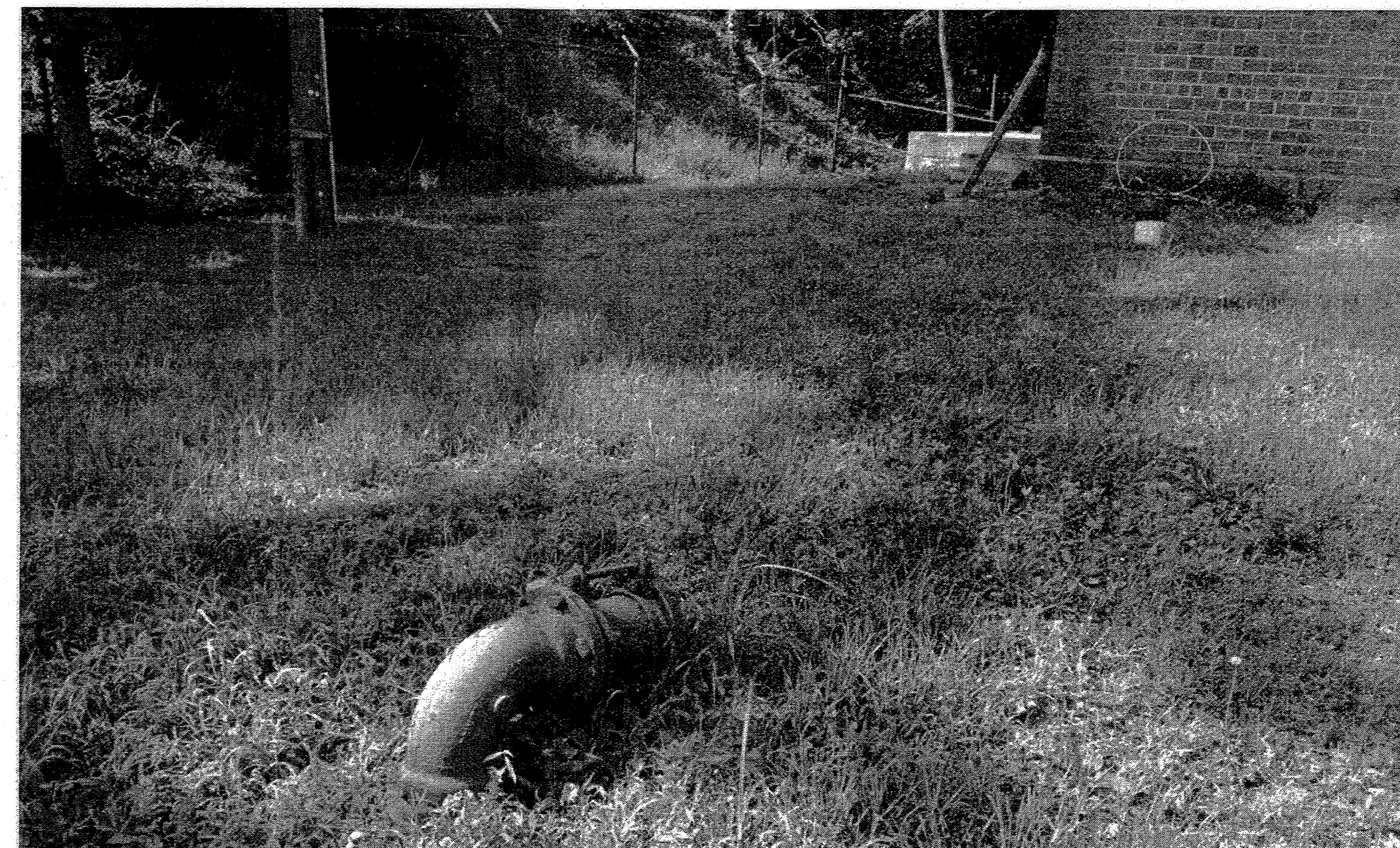
2 D-3 DEMOLISH 6" BYPASS CONNECTION ②④
