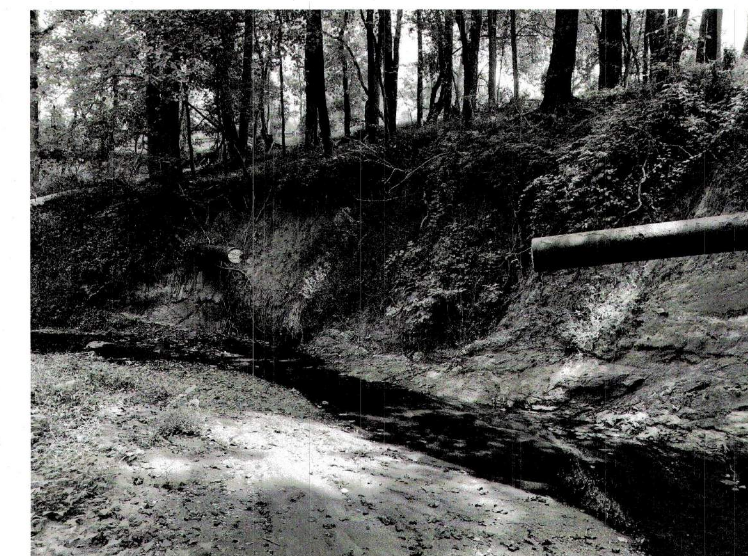
3 PHOTO OF ABANDONED PIPES TO CUT AND CAP AT STREAMBANK SCALE: NO SCALE
