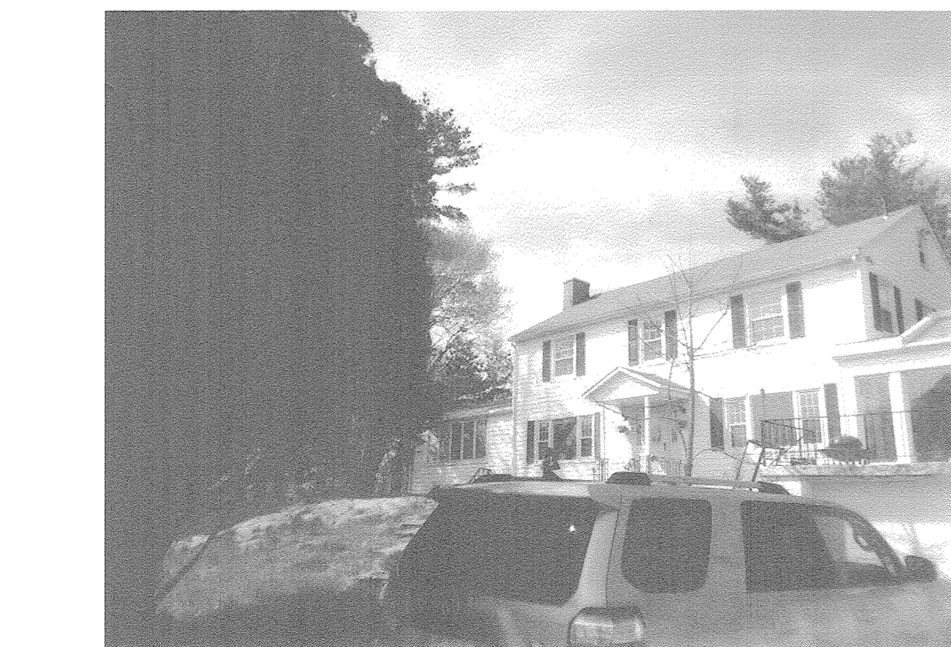
EXISTING HOUSE PHOTO NOT TO SCALE
