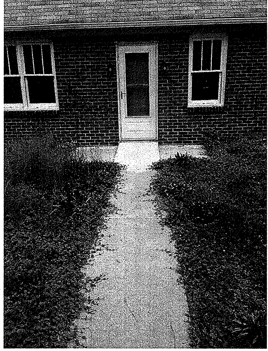
EXISTING HANDICAP ACCESS
