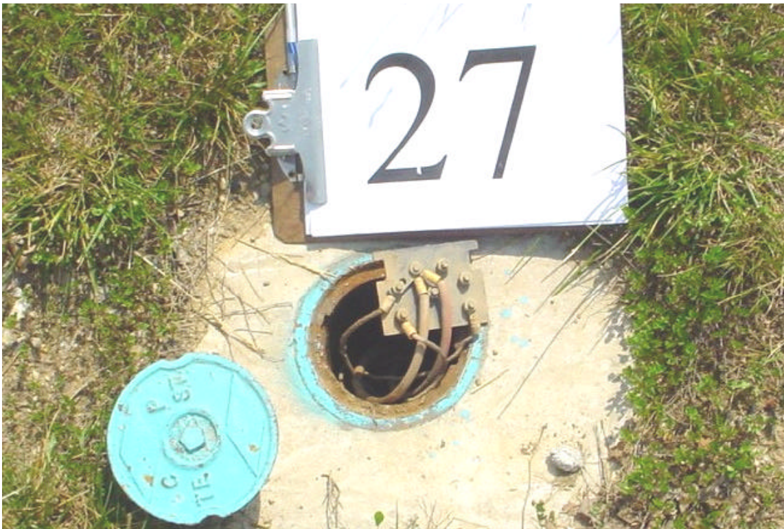
Figure 53 - Test Station #27, close-up
