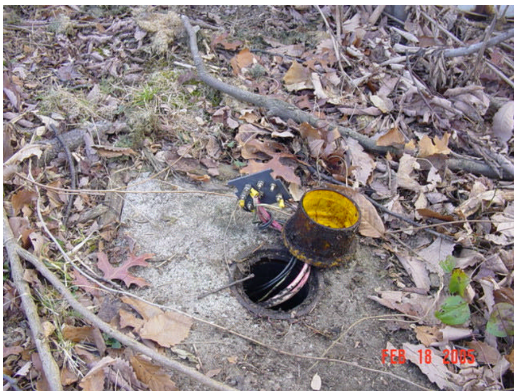
Figure 174 – Test Station 26 close up
