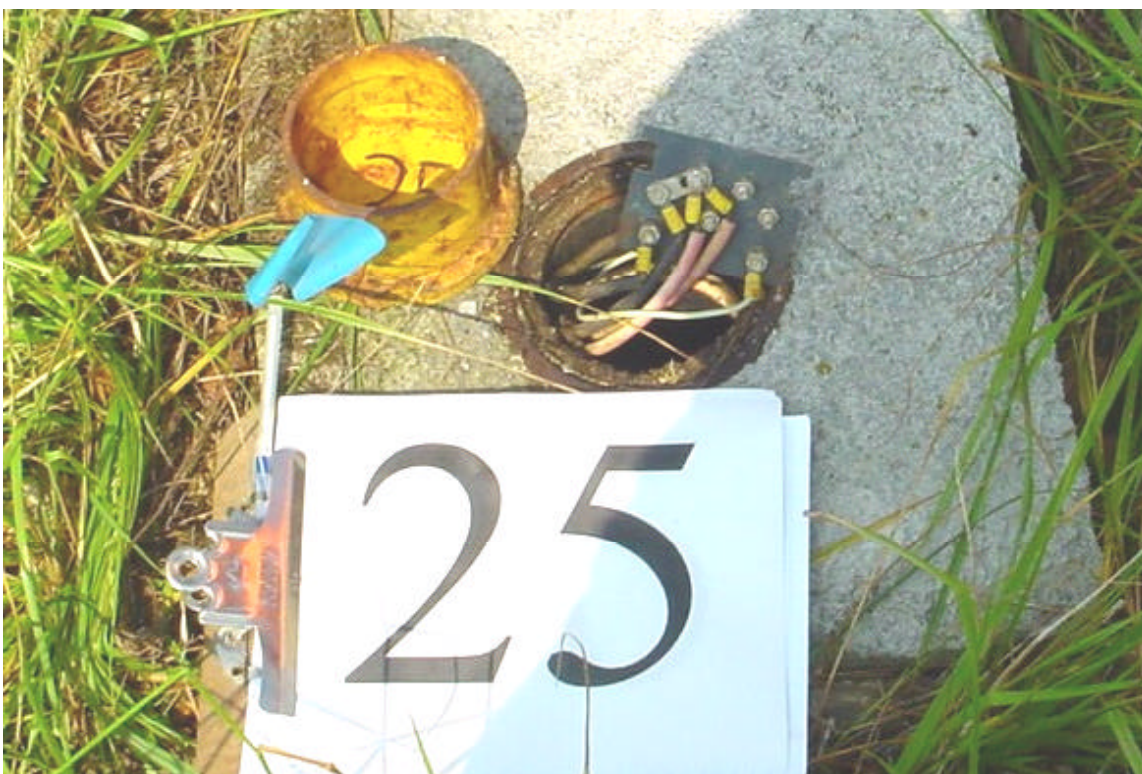
Figure 49 - Test Station #25, close-up
