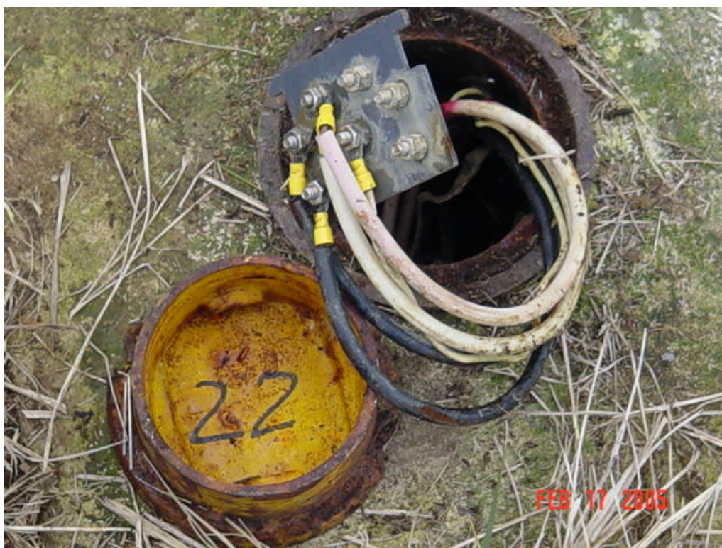
Figure 166 – Test Station 22 close up
