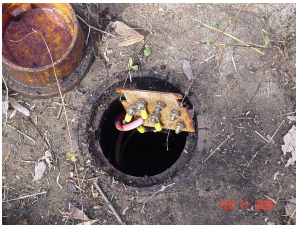
Figure 164 – Test Station 21 close up
