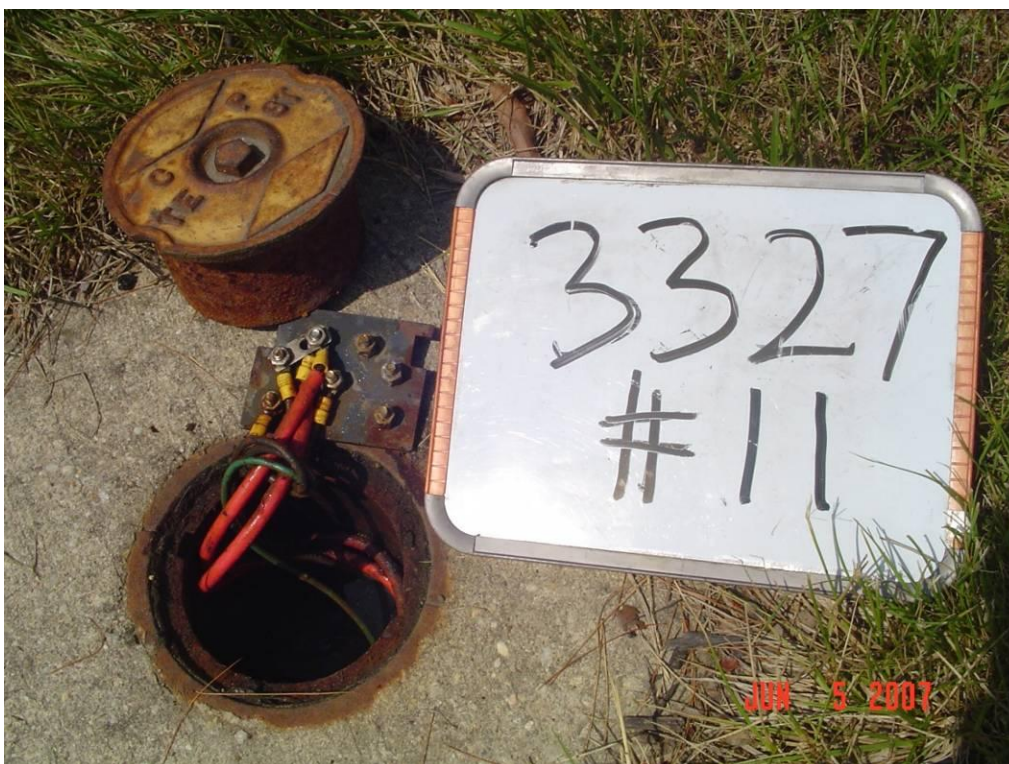
Figure 142 – Test Station 11 close up
