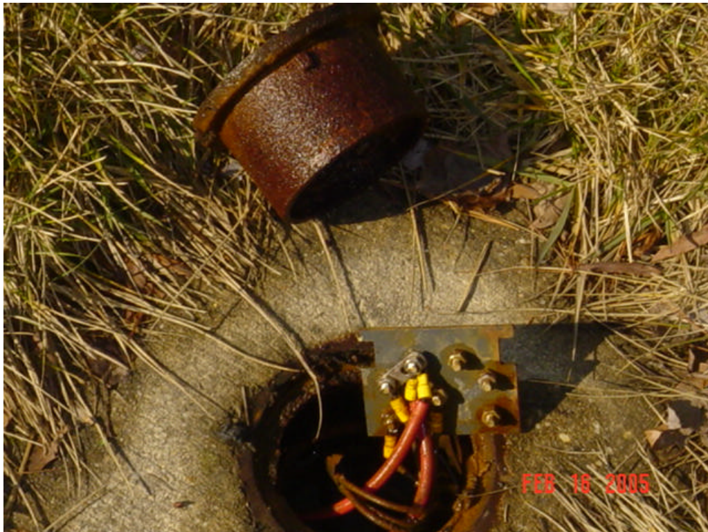
Figure 146 – Test Station 10 close up
