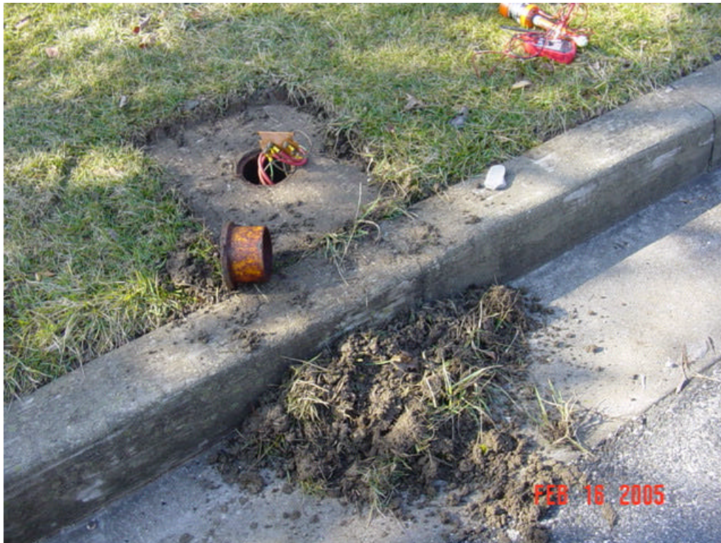
Figure 144 – Test Station 9 close up
