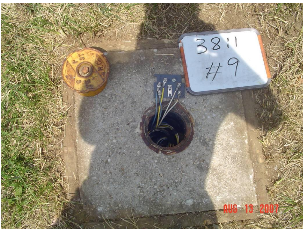
Figure 201 - Test Station 3811-9 close-up
