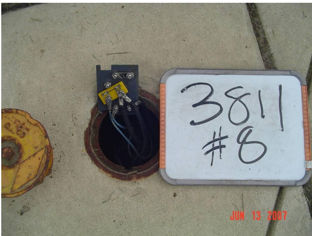
Figure 199 - Test Station 3811-8 close-up
