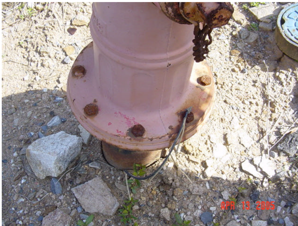
Figure 229 - Test Station 3480-3 close-up
