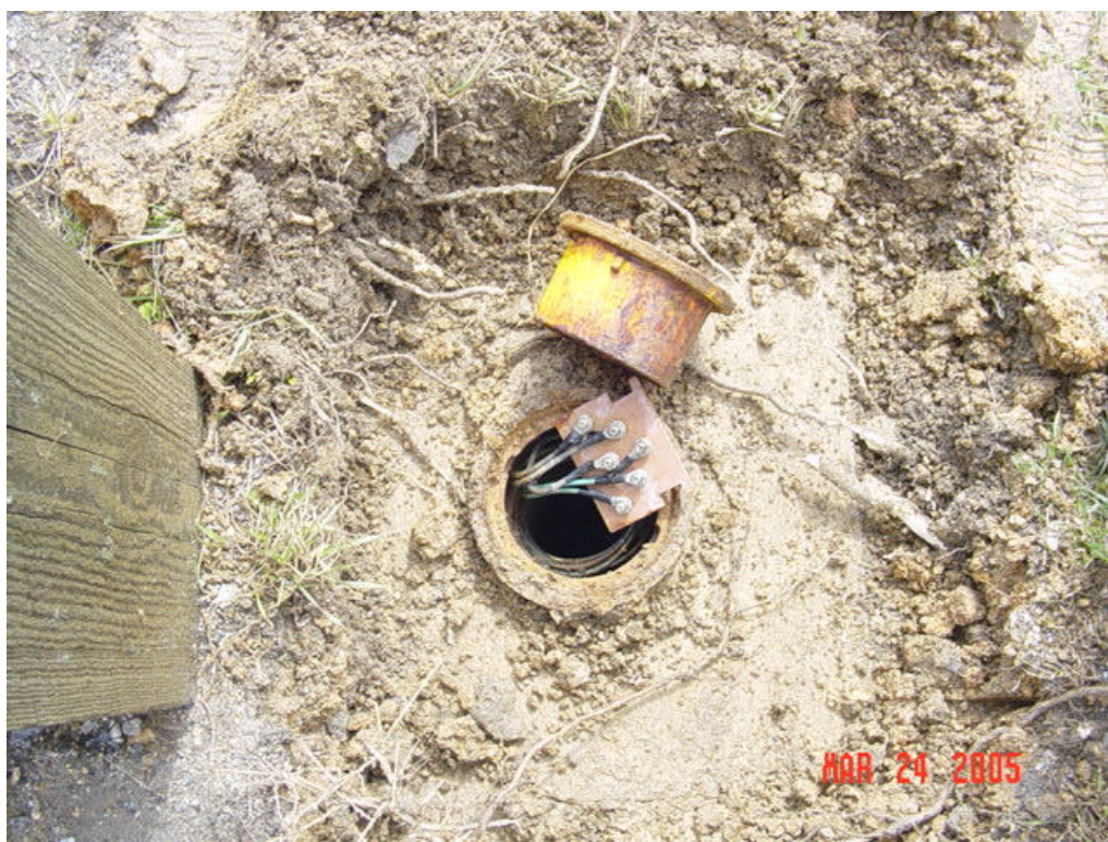
Figure 121 - Test Station 3231-1 close-up
