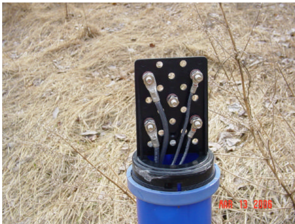
Figure 8 – Test Station 3 close-up
