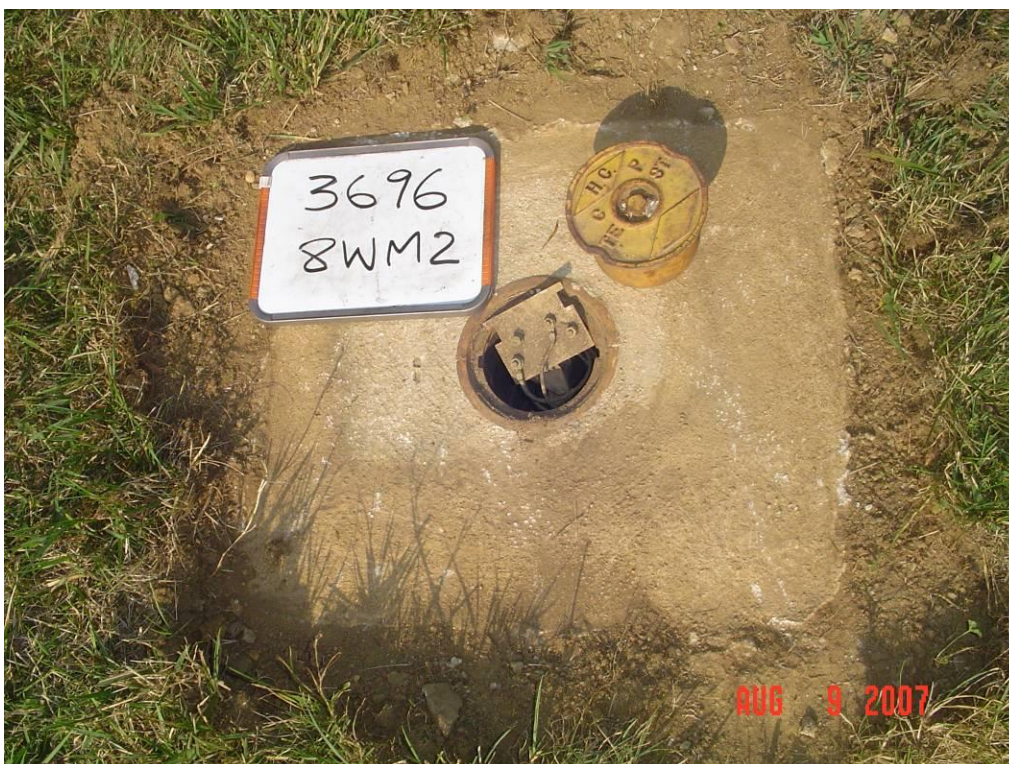
Figure 7 - Test Station 8WM2 close-up
