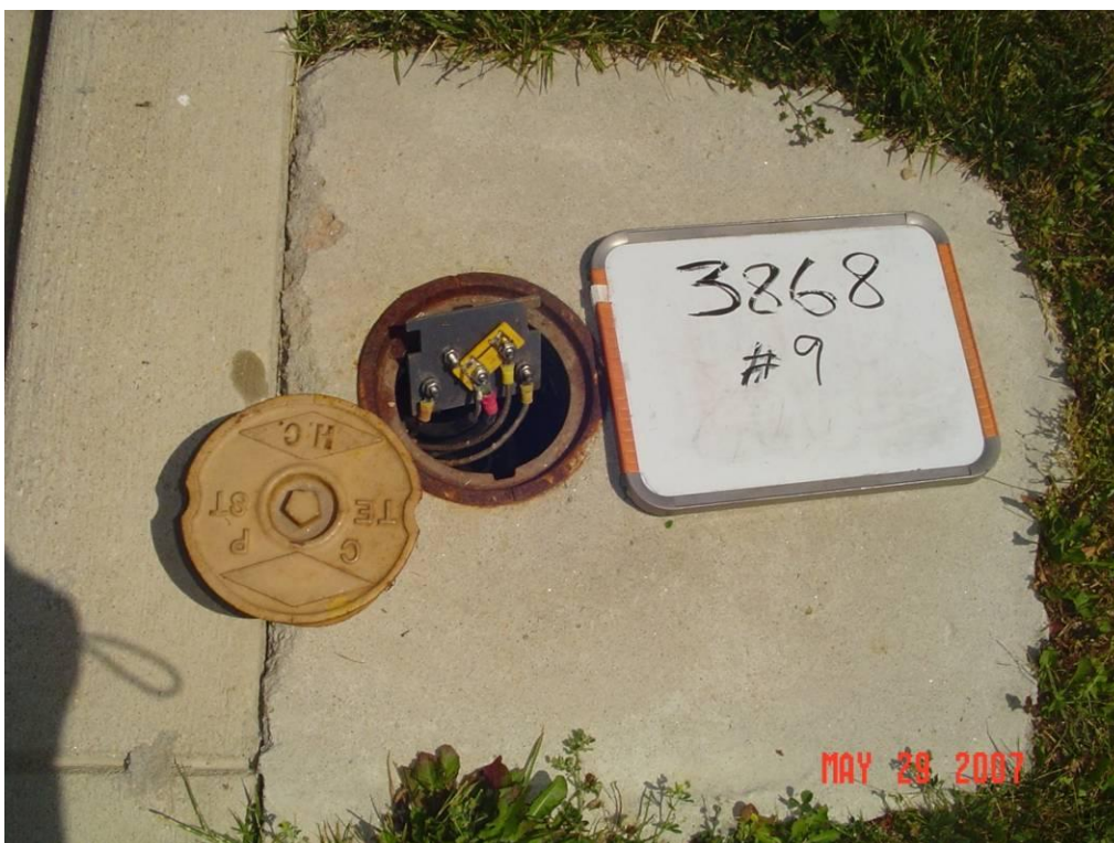
Figure 91 – Test Station 9 close up
