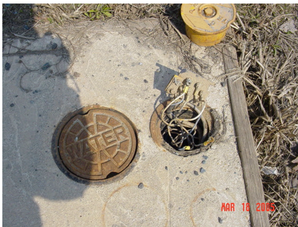
Figure 103 – Test Station 8 close up
