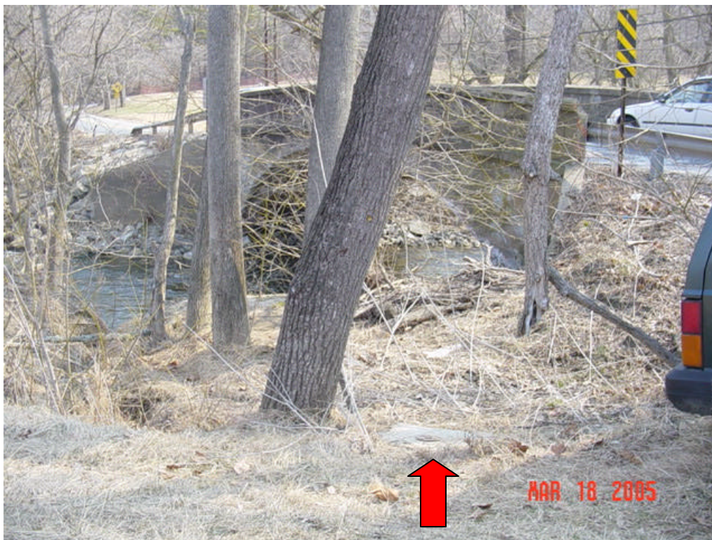
Figure 96 – Location of Test Station 5 - Old Columbia Road and Middle Patuxent River
