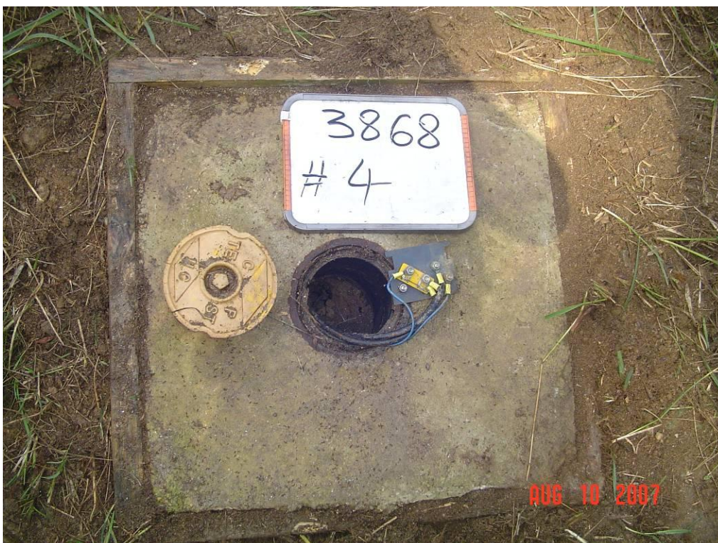
Figure 81 – Test Station 4 close up
