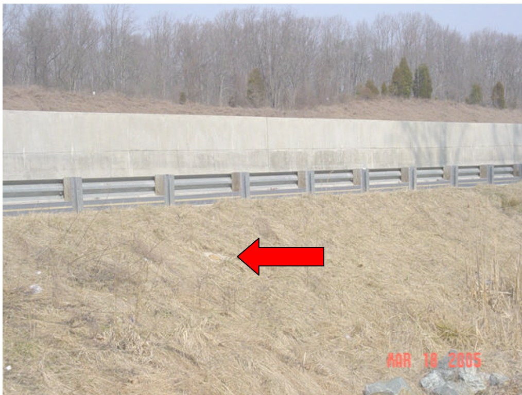
Figure 94 – Location of Test Station 4 - Old Columbia Road
