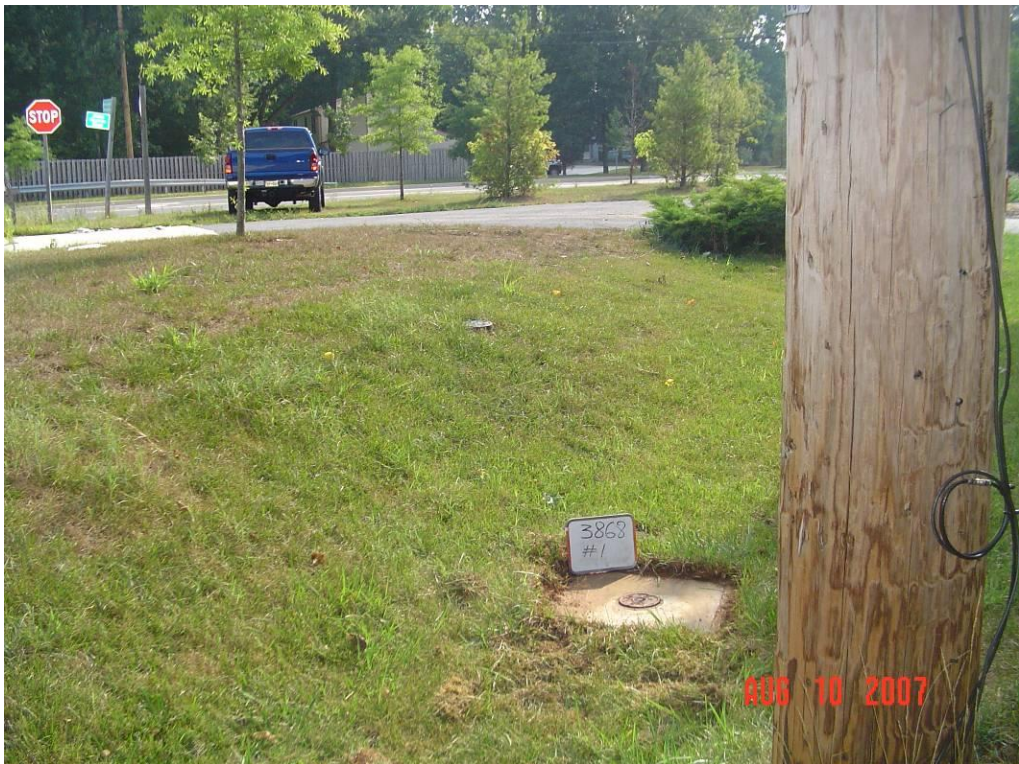
Figure 72 – Location of Test Station 1 - Hammond Parkway & Johns Hopkins Road
