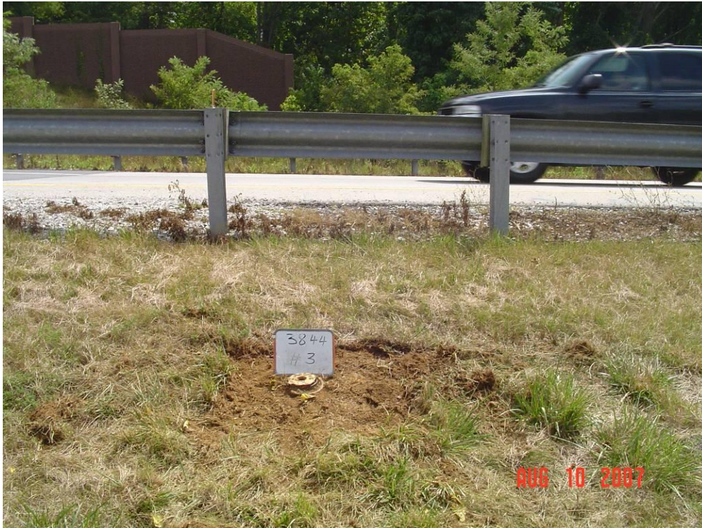
Figure 65 – General area of Test Station 3844-3
