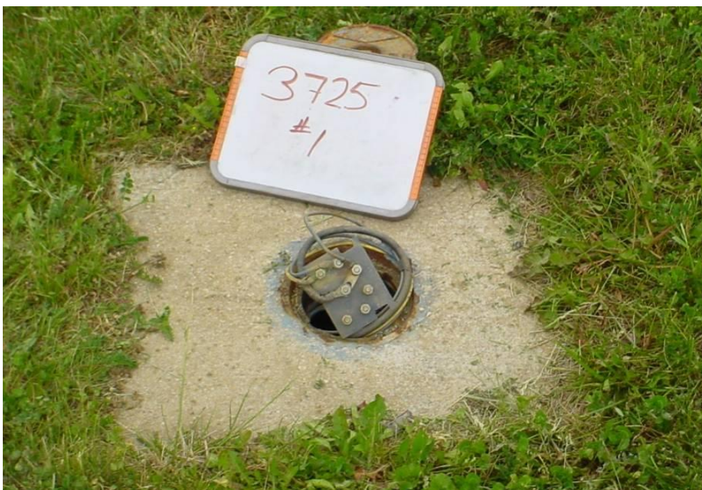
Figure 38 - Test Station 3725-1 close-up
