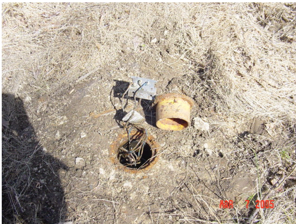
Figure 19 – Test Station 12GS6 close-up
