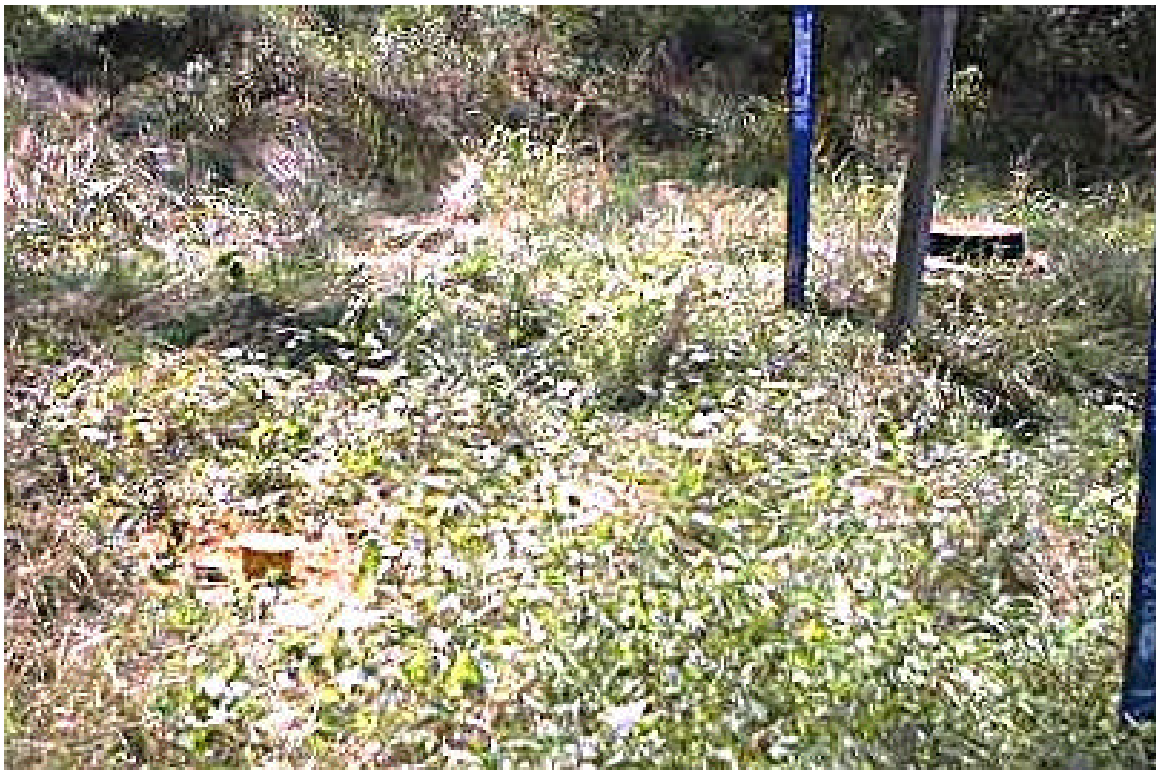
Figure 34 - Test station 12GS4
