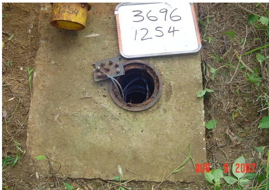
Figure 15 - Test Station 12GS4 close-up
