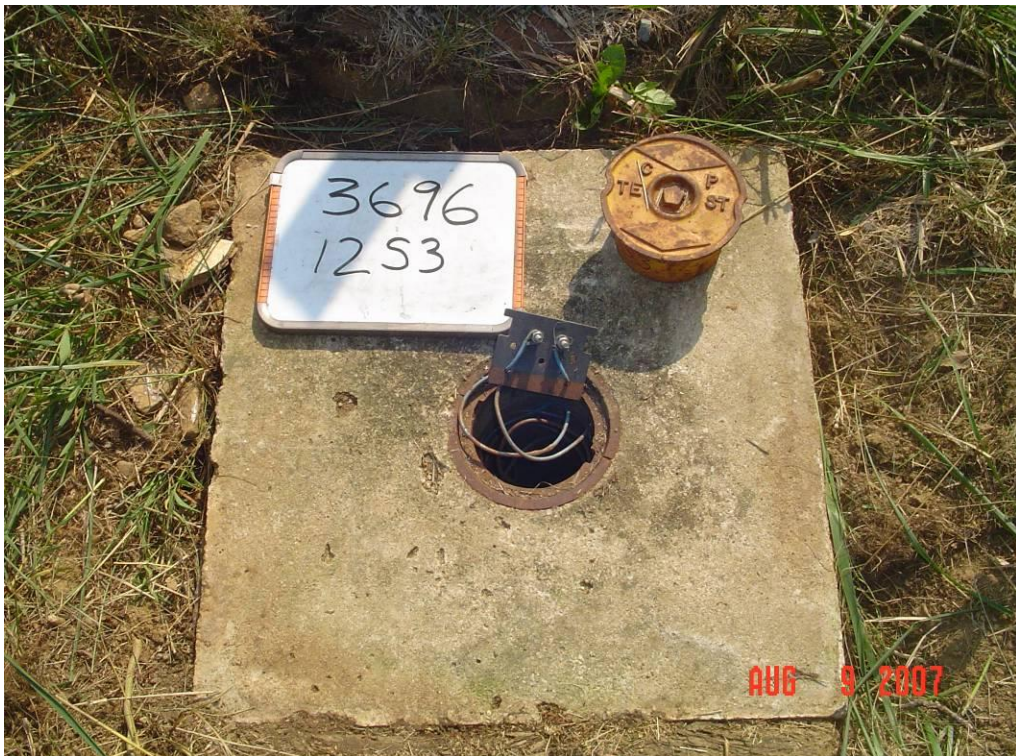
Figure 13 - Test Station 12GS3 close-up
