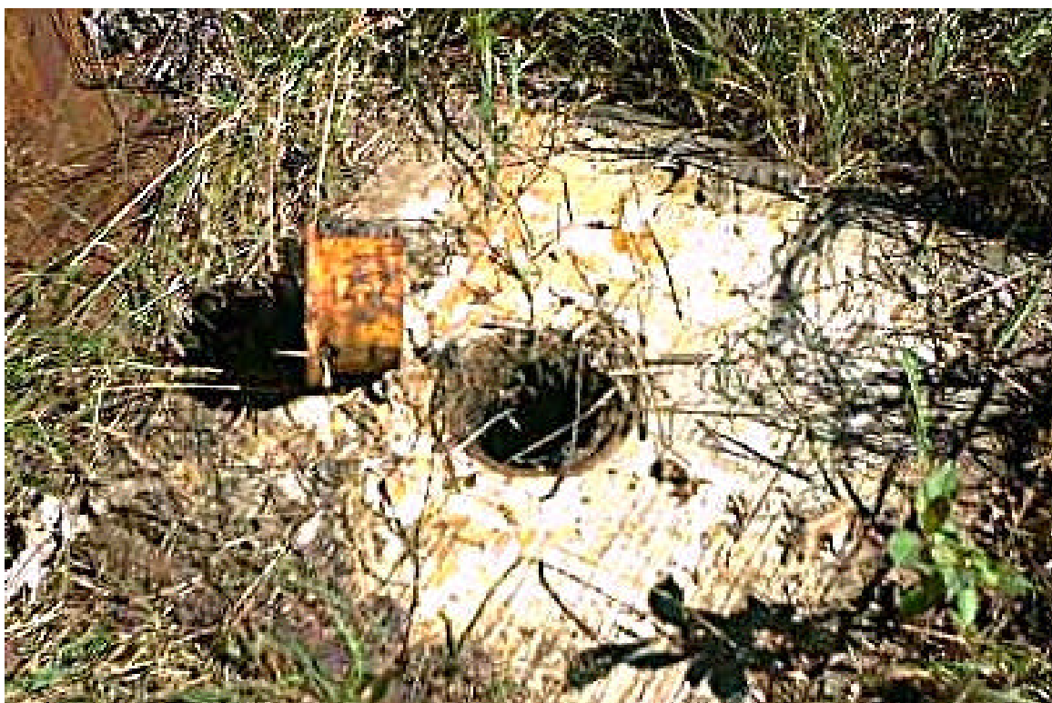
Figure 31 - Test station 12GS2, close-up
