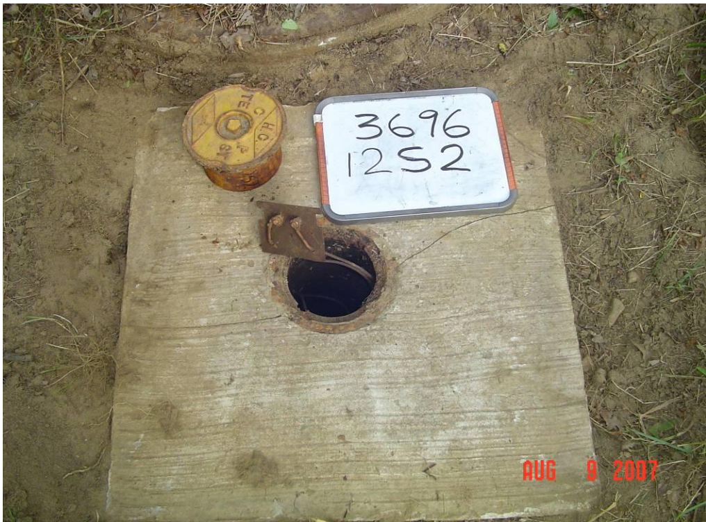
Figure 11 - Test Station 12GS2 close-up
