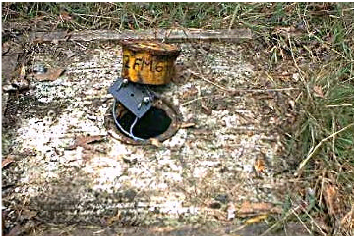
Figure 23 - Test station 12FM6, close-up
