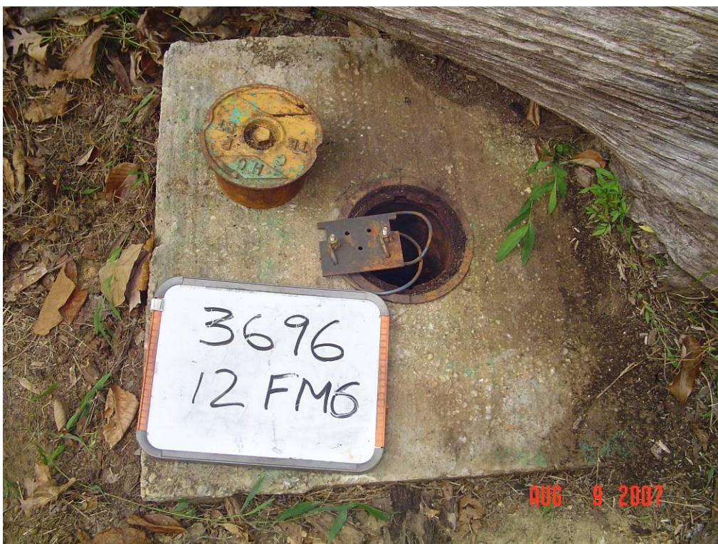
Figure 27 -Test Station 12FM6 close-up
