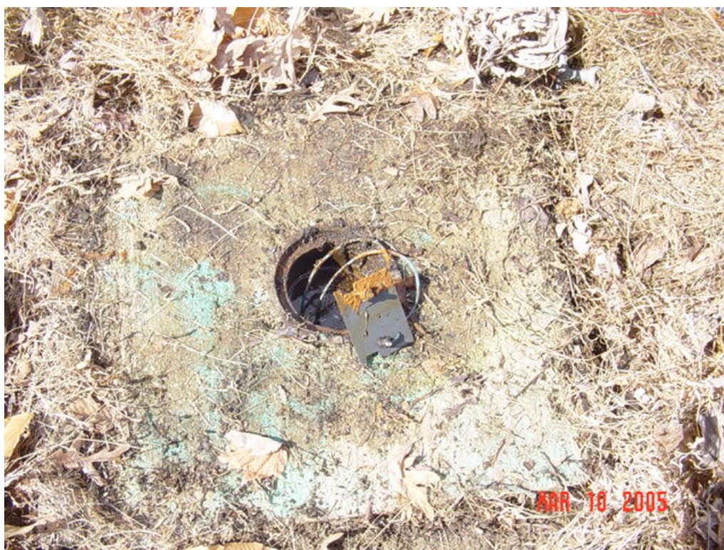
Figure 29 -Test Station 12FM6 close-up
