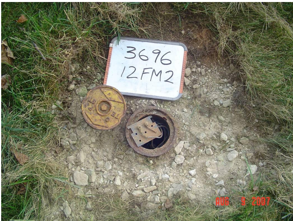
Figure 21 - Test Station 12FM2 close-up
