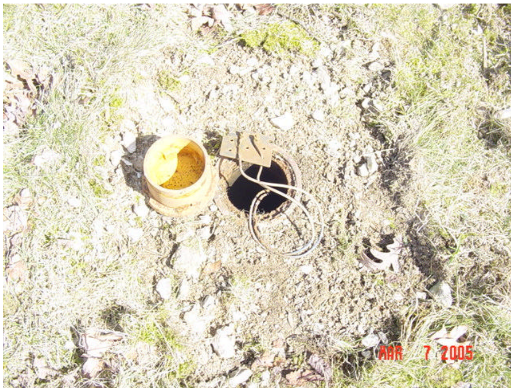
Figure 23 - Test Station 12FM2 close-up
