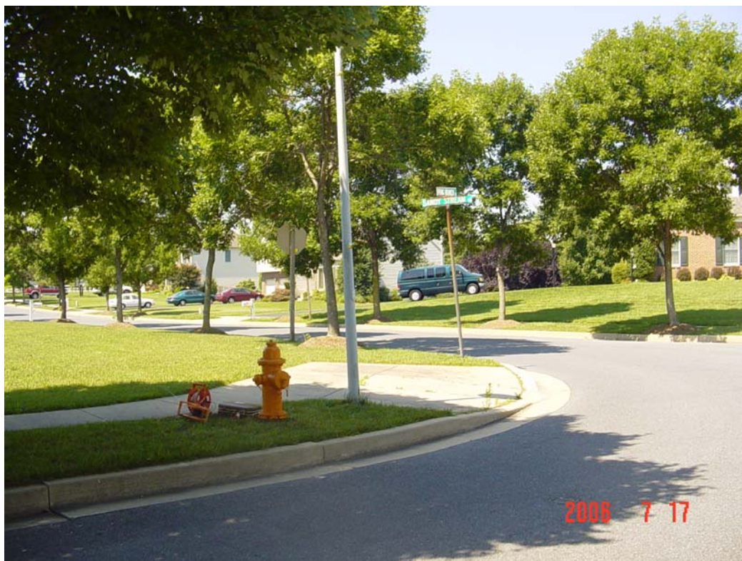
Figure 82 - Measuring stray currents near the Sandy Stream Road and Spring Branch Court intersection
