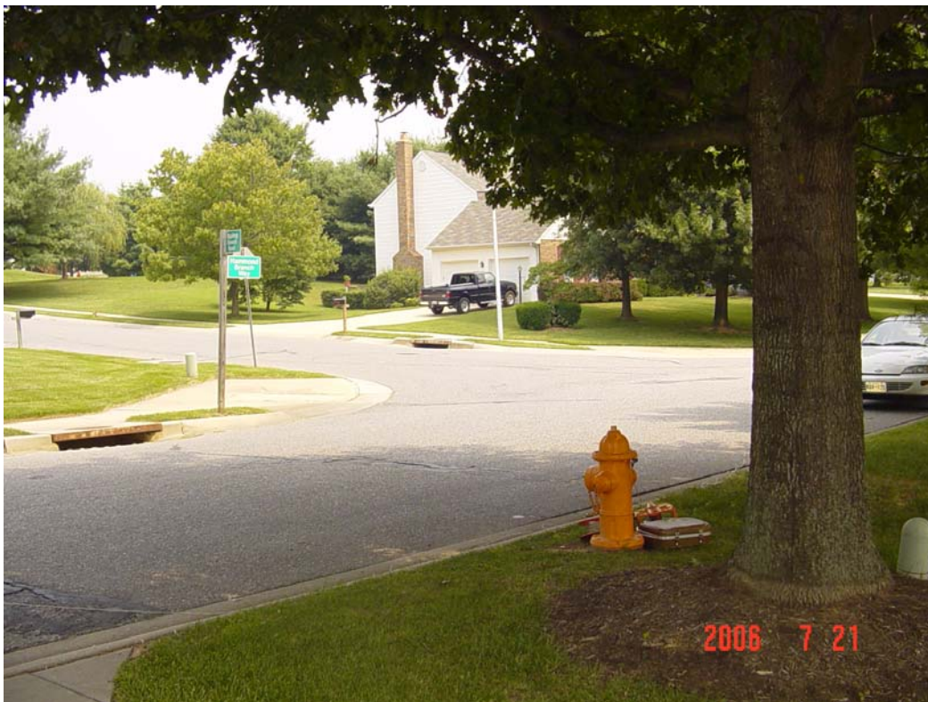
Figure 88 – Measuring stray currents near the Rippling Branch Rd. and Hammond Branch Way intersection
