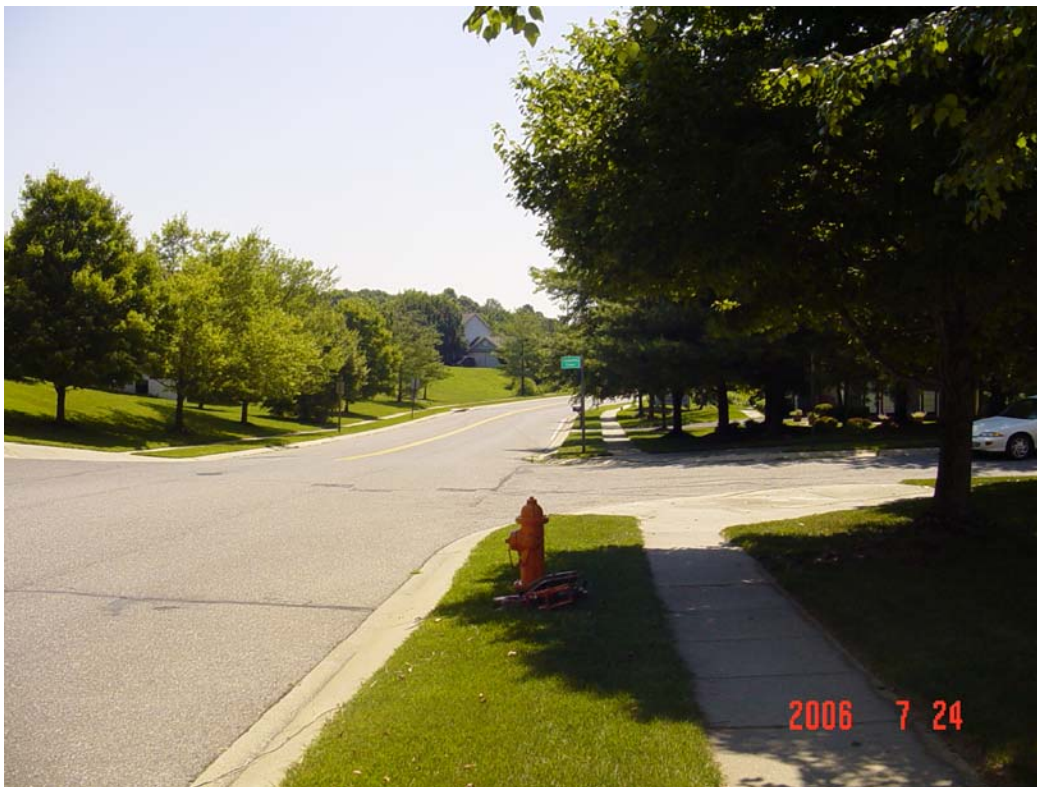
Figure 94 – Measuring stray currents near the Hammond Branch Way and Crest Road intersection
