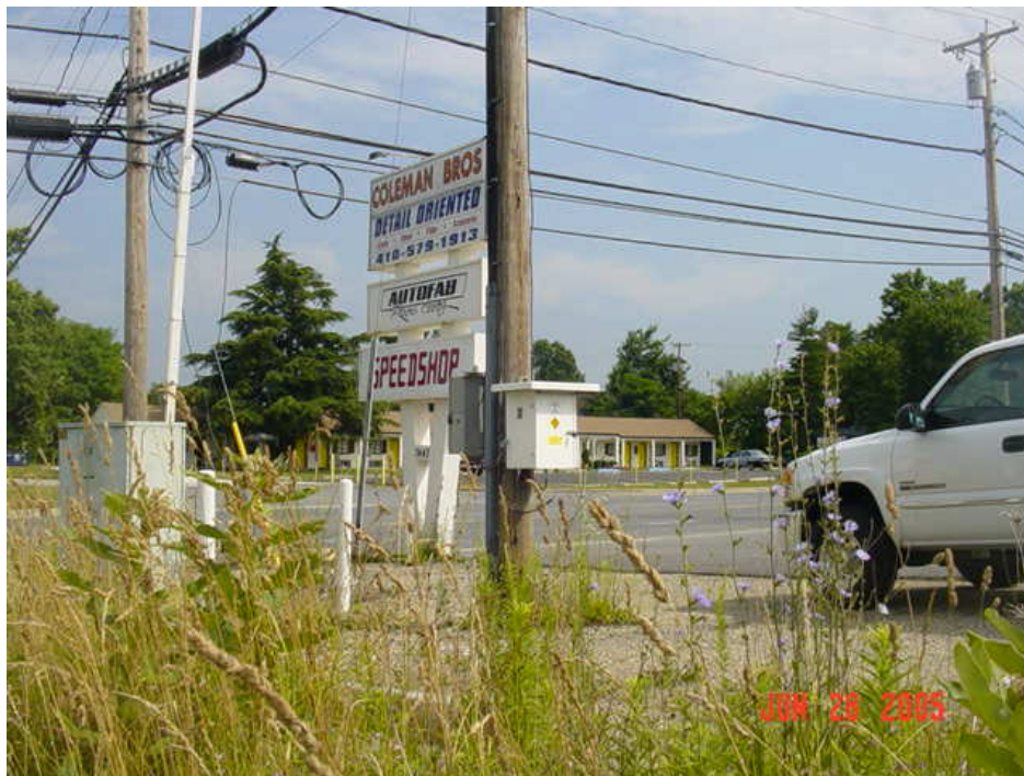
Figure 17 - Impressed Current Rectifier BGE5
