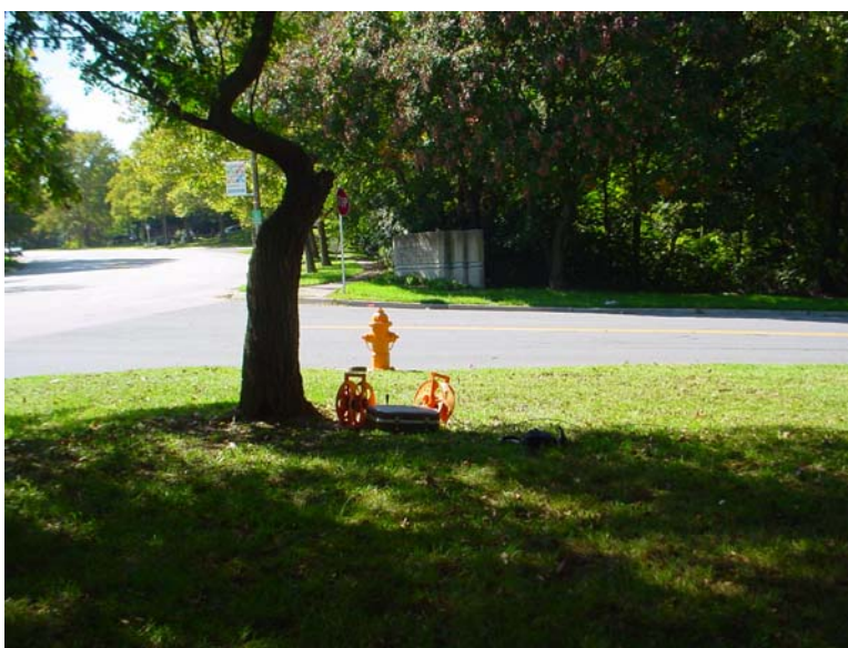
Figure 66 – Measuring stray currents at the location Twin Knolls Road 3
