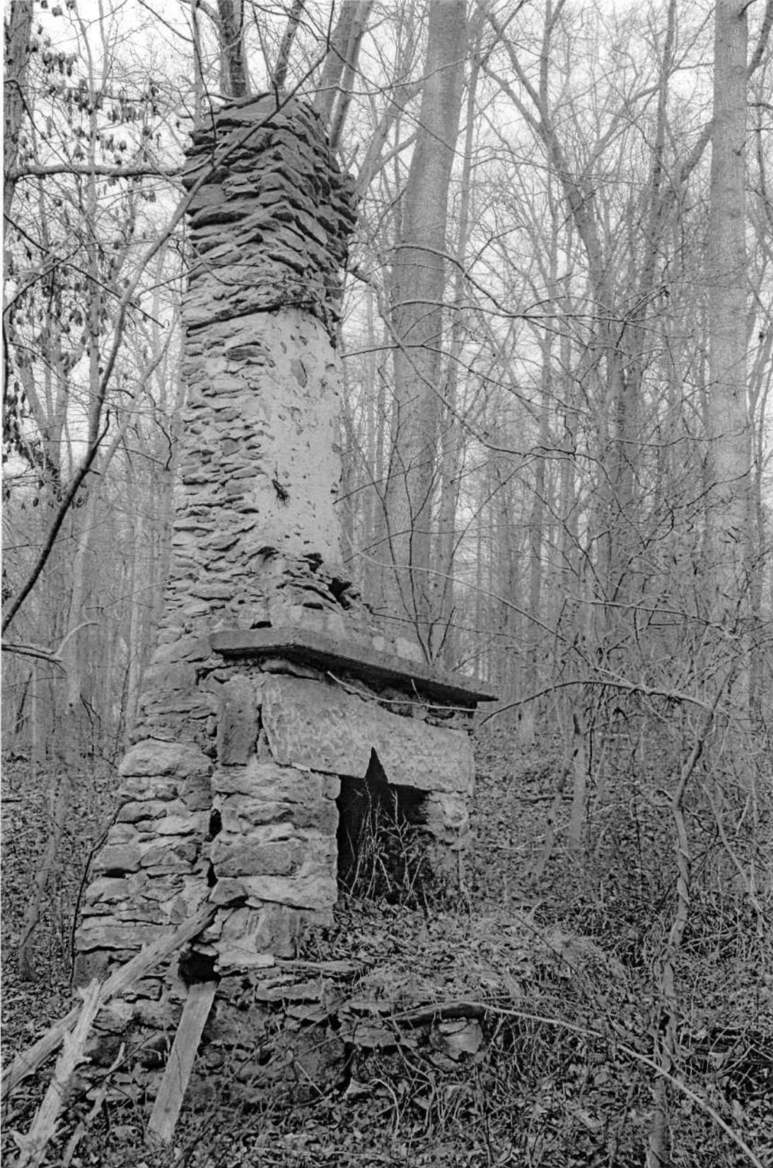
HO-931 Roxbury Road Boy Scout Cabin Old Roxbury Road Chimney from southwest Ken Short, December 2006 2/2
