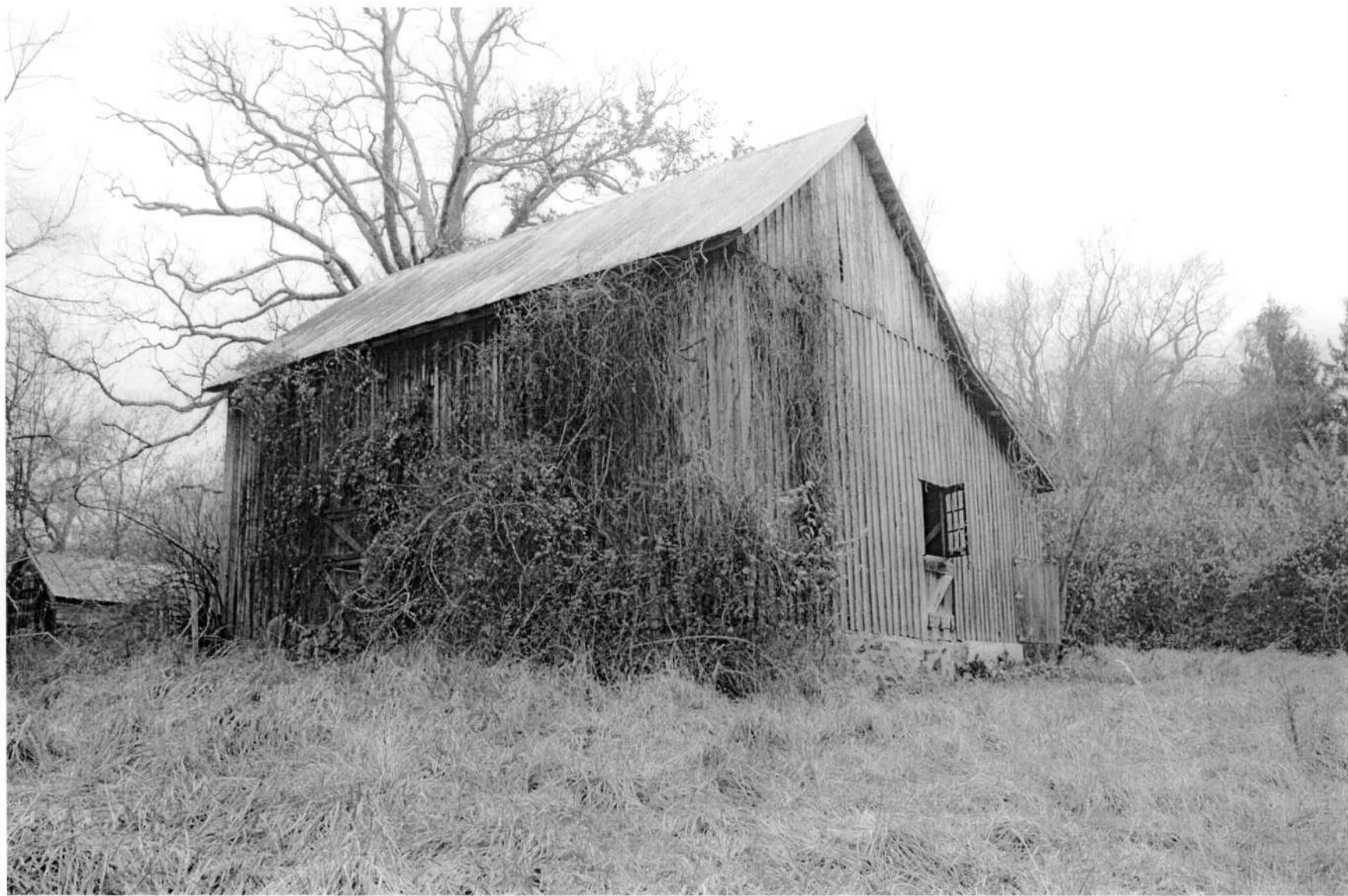
HO-928 Manatee-Thompson Farm 5710 Trotter Road Barn, south & east elevations Ken Short, December 2006 5/5
