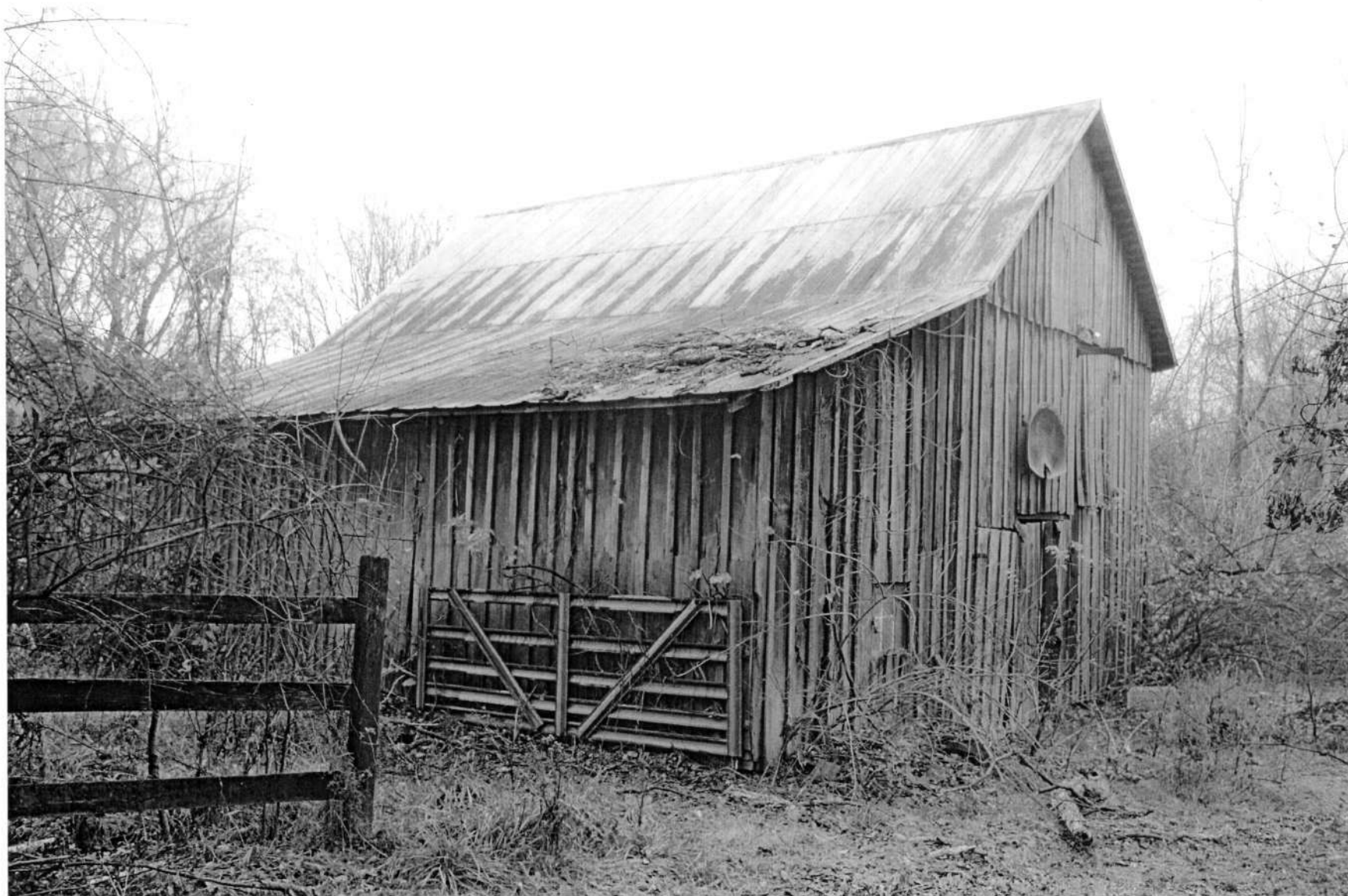
HO-928 Manatee-Thompson Farm 5710 Trotter Road Barn, north & west elevations Ken Short, December 2006 4/5
