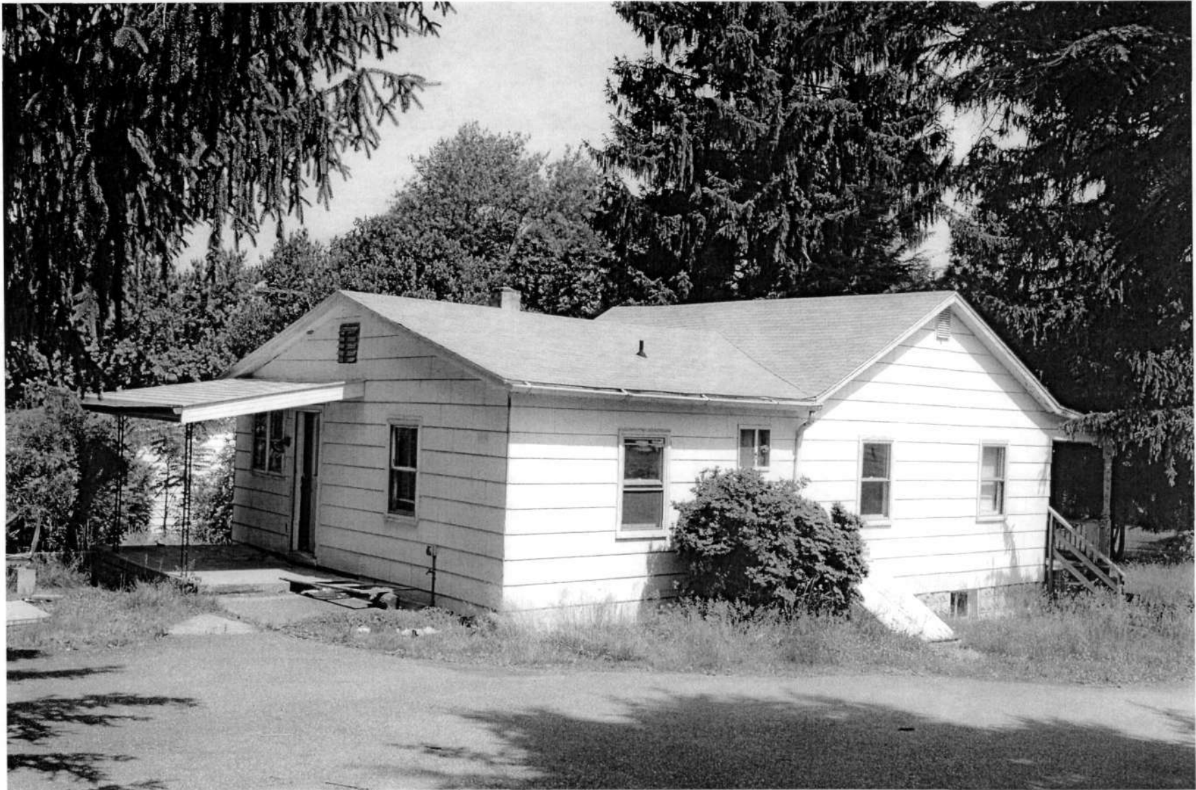
HO-912 Seicke-Wood House 9577 Old Annapolis Road Southwest & southeast elevations Ken Short, May 2006 3/4
