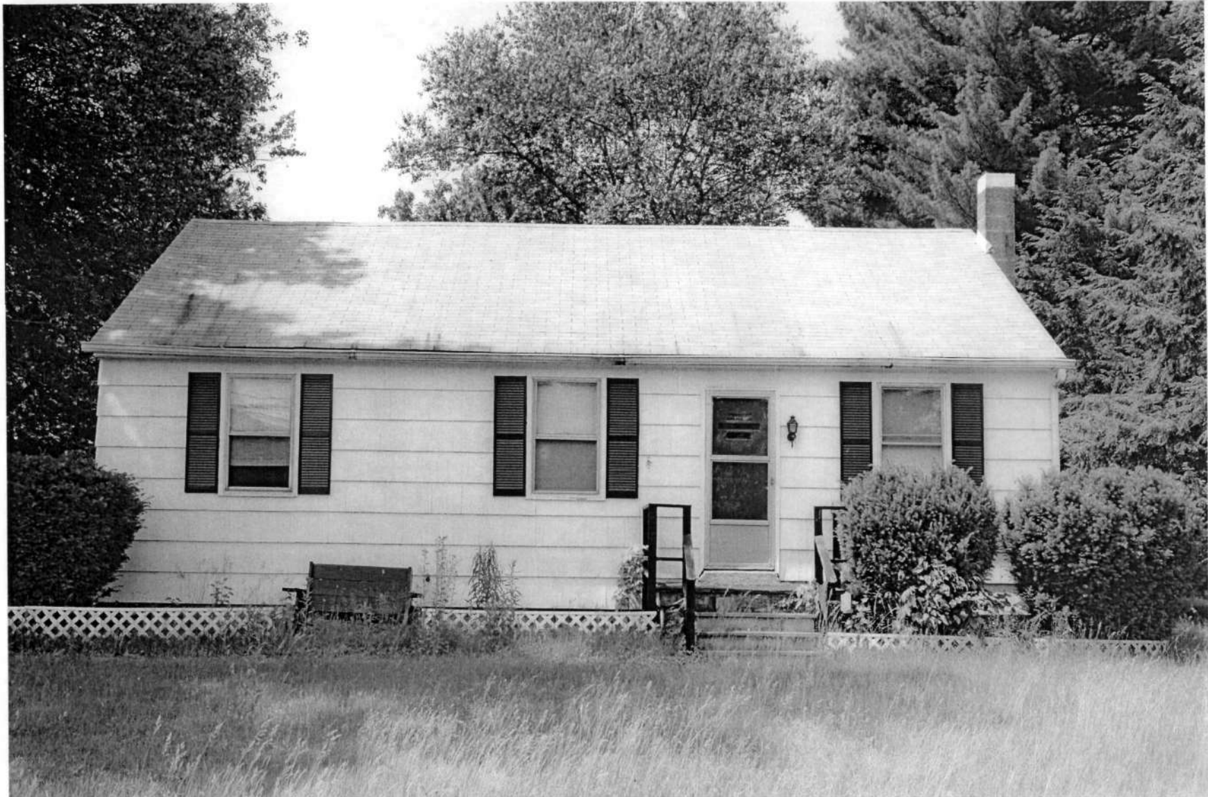
HO-911 Seicke-Ketterman House 9571 Old Annapolis Road Northeast elevation Ken Short, May 2006 1/3
