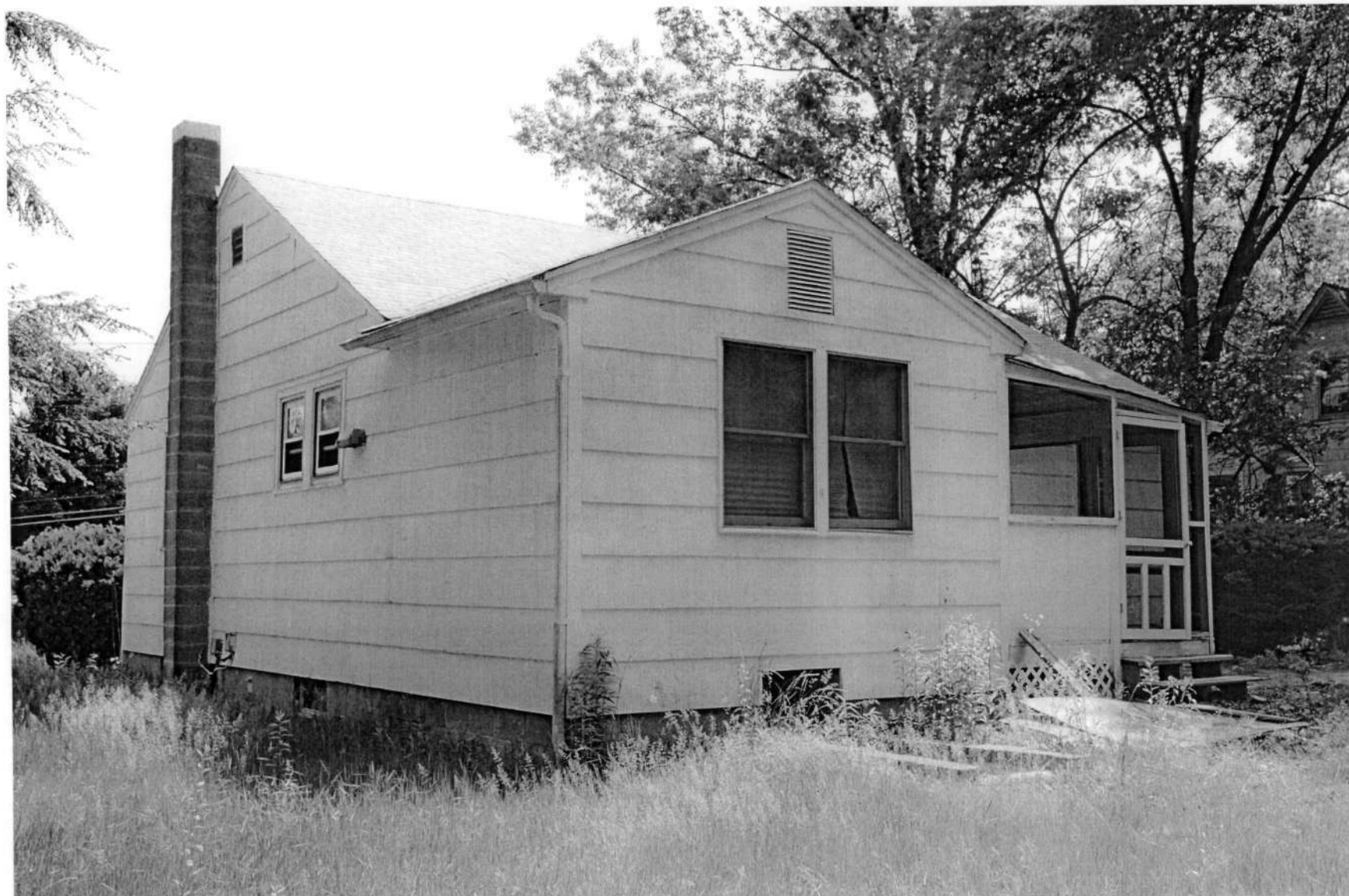
HO-911 Seicke-Ketterman House 9571 Old Annapolis Road Northwest & southwest elevations Ken Short, May 2006 2/3
