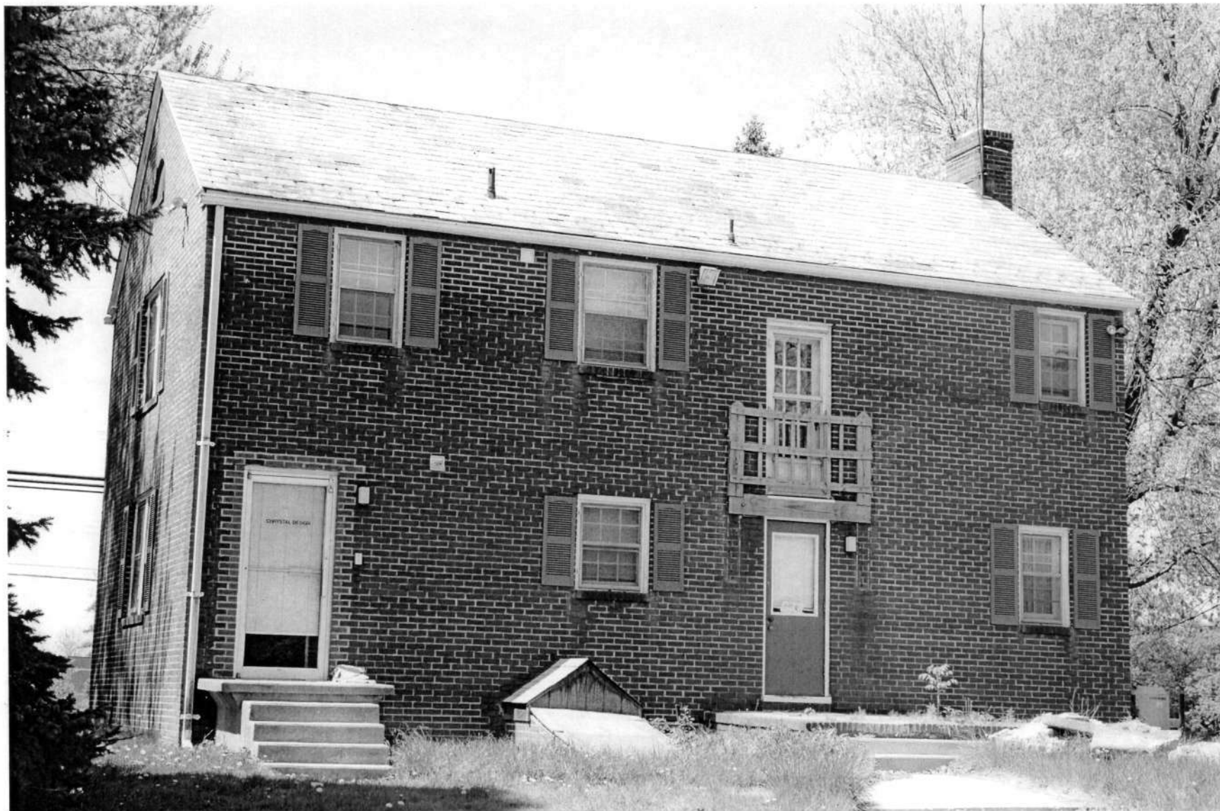
HO-0905 Earl & Evelyn Hemminger House 4253 Montgomery Road, House-east elevation Ken Short, April 2006 2/6
