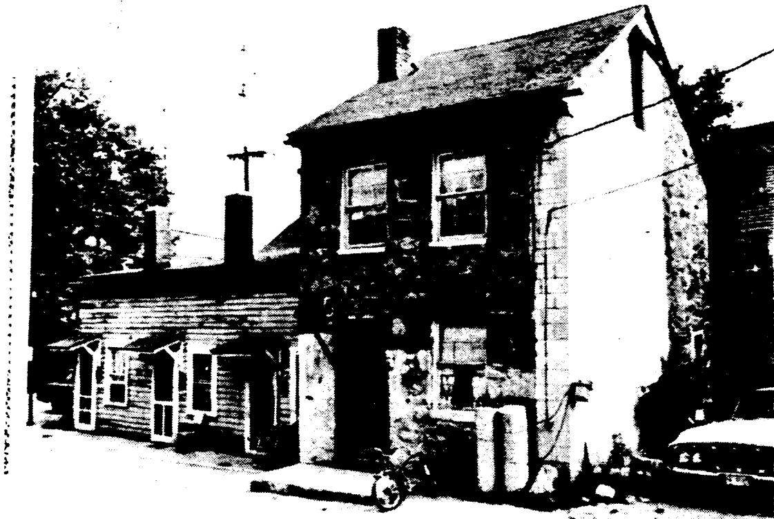
FIRST COUNTY SEAT--The stone building is the original County Court House, which served as the first County seat from at least 1840 to 1843. A resolution concerning its preservation together with the Howard District Jail was introduced at Monday's night session of the County Council.
