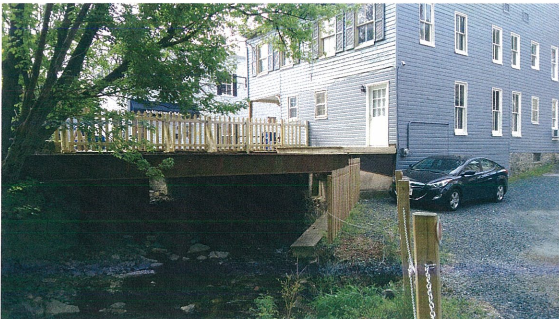
Stream view under deck
