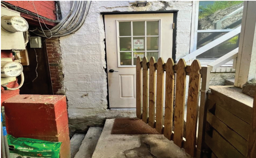
Photo Four Caption: 2nd floor entrance 04/29/2024 ( east side )
