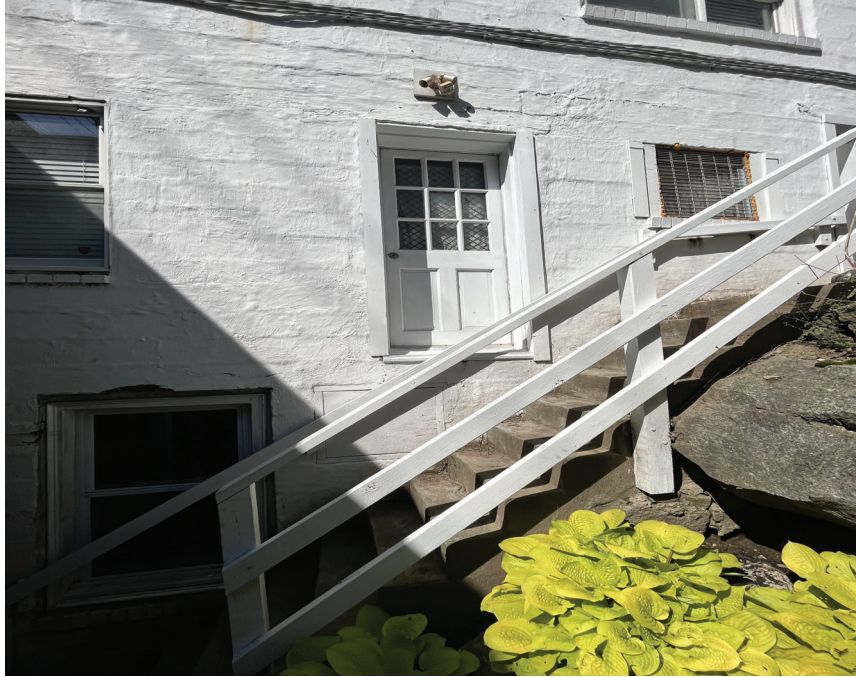
Photo Three Caption: 3rd floor entrance 04/29/2024 (north east side of building)
